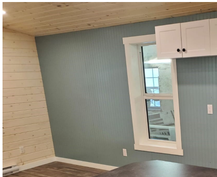
Painted Paneling Wall, White- washed Pine Wall, & Clear Pine
